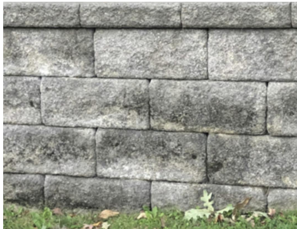
BLOCK RETAINING WALL 8" INTERLOCKING BLOCKS
